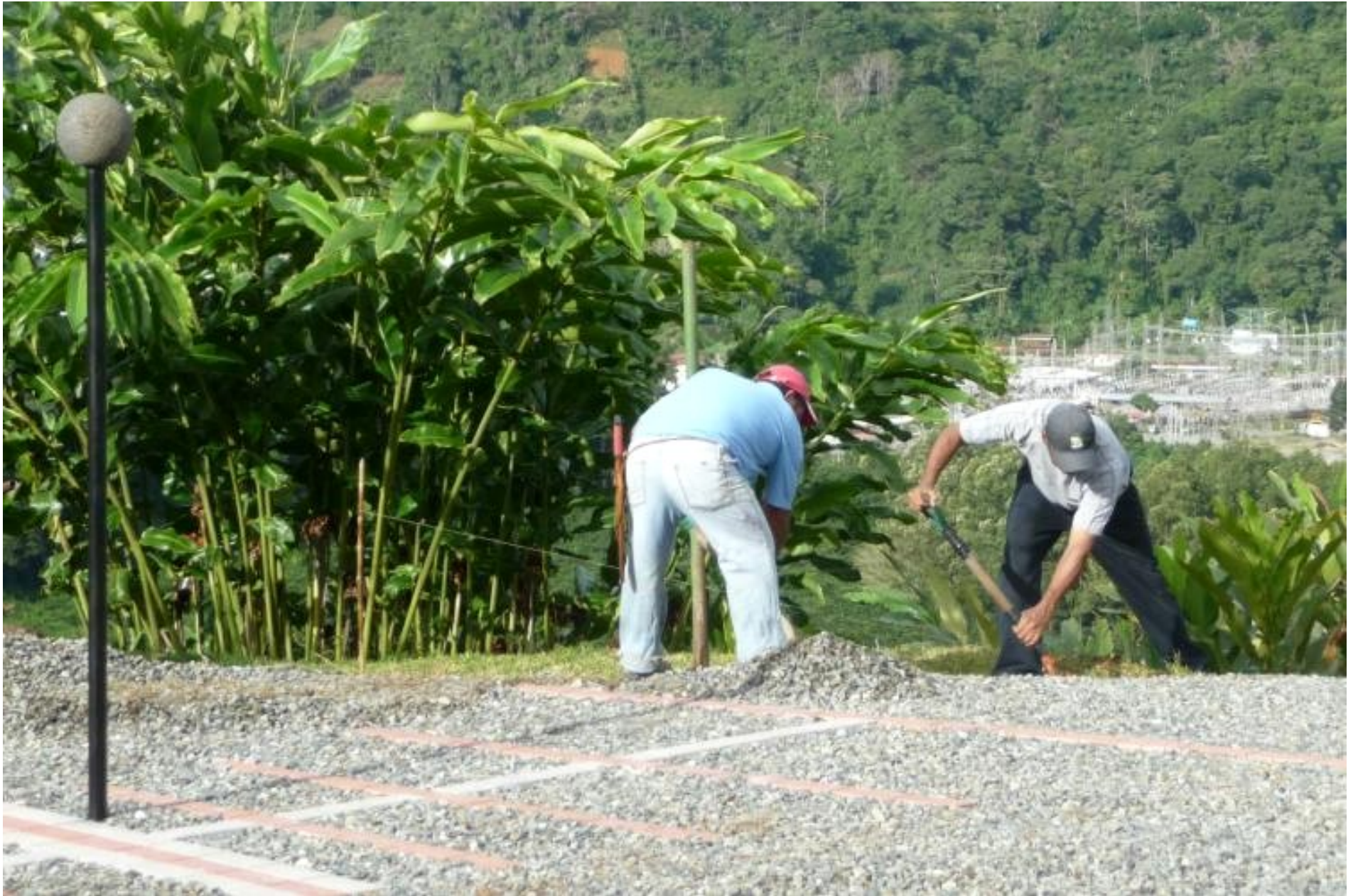
The excavation begins
