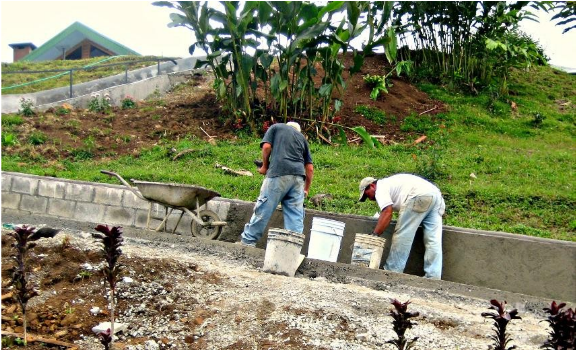
Covering the block walls with a cement mixture.
