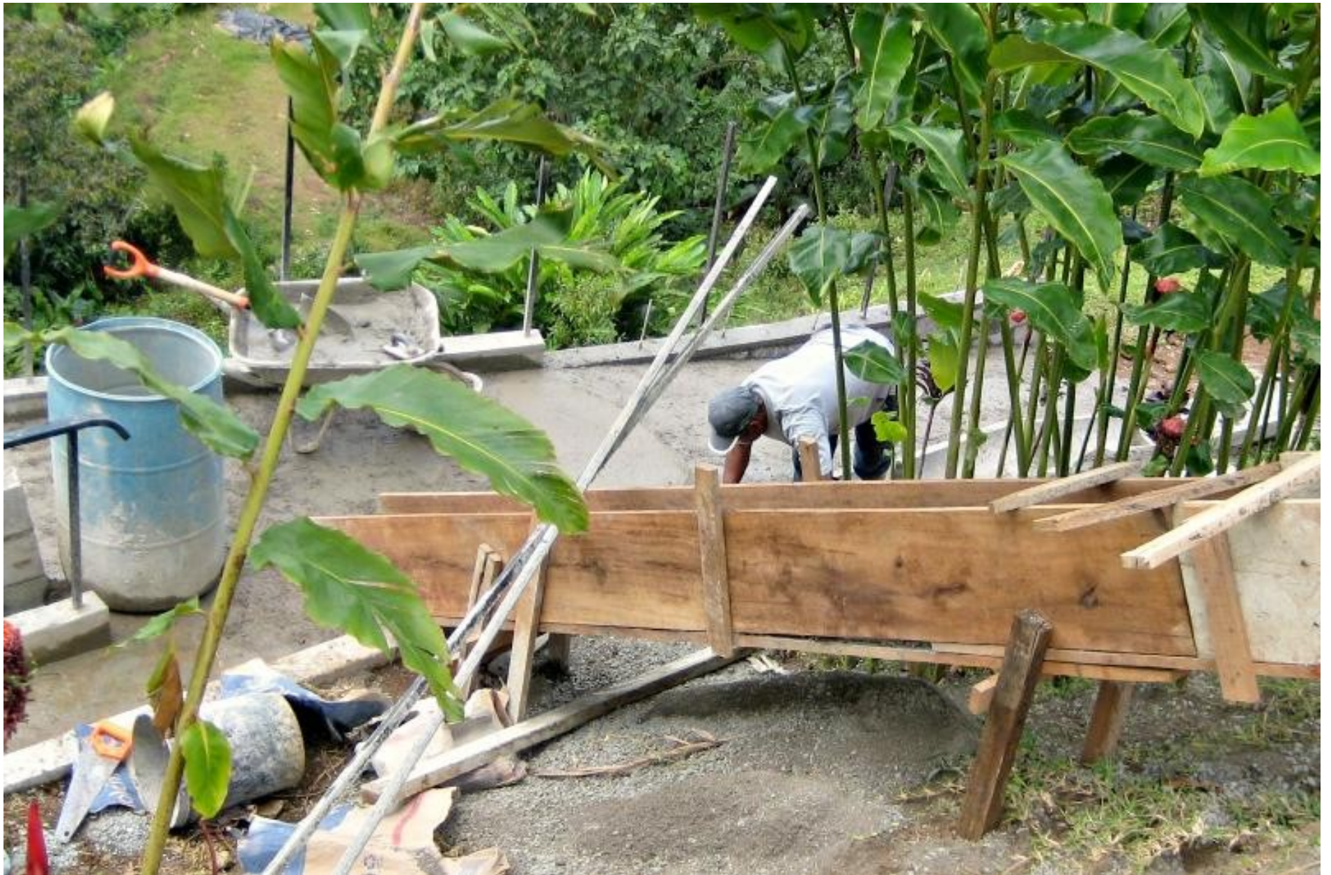
Building a ramp to access the new north sendero.
